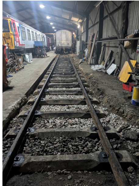
(Above) The Loco Road in the Restoration Shed after relaying
