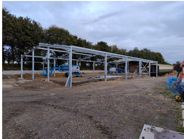
The framework for the new Heritage Centre before the cladding was applied
