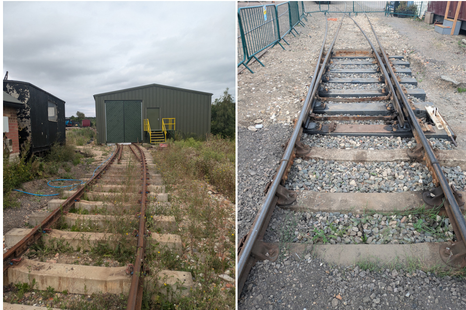
(Left) the line leading down to the Exhibition Hall, and (right) the new points installed on the back road (both Josh Fortescue)
