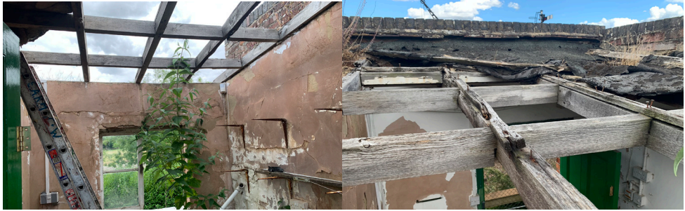
▲ Two views of the Lamp Room - showing the poor condition and missing roof.
