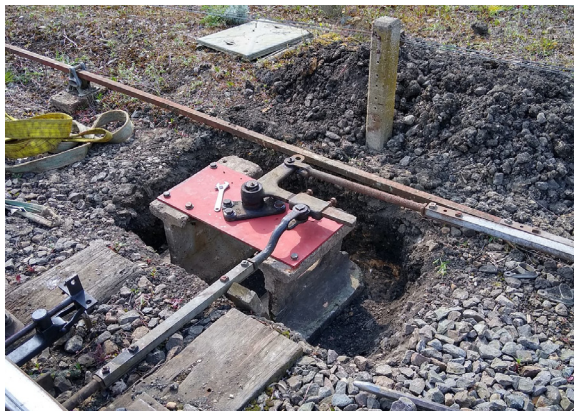
► One of the new crank beds installed at the Museum - Jack Plumb
