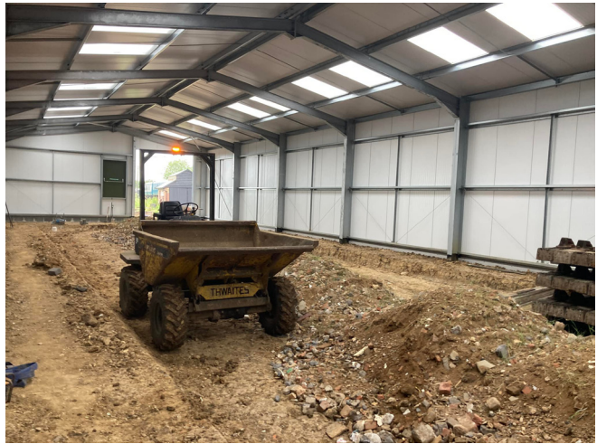
▲ Groundworks on-going in the Exhibition Hall to prepare for the track and final floor on 6 June 2022 - Tim Rice.
