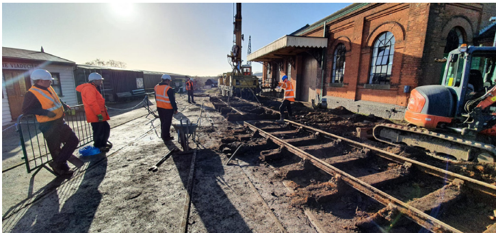
◀ The PWay gang removing the track panels near the Goods Shed on 9th January 2022 - Mike Bradley.
