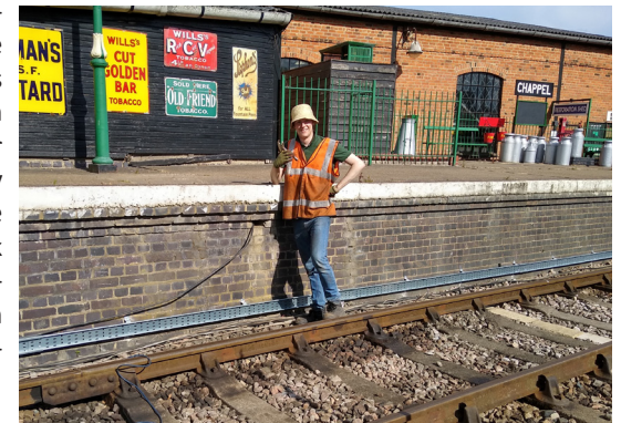
▲ Jack installing a cable tray on Platform 3 on 22nd June 2020 Elsewhere, a cable tray has been installed along the length of the Platform 3 wall, tidying up the cables which previously hung loosely along the platform wall. The signal gantry also got a clean and the final few painting jobs
