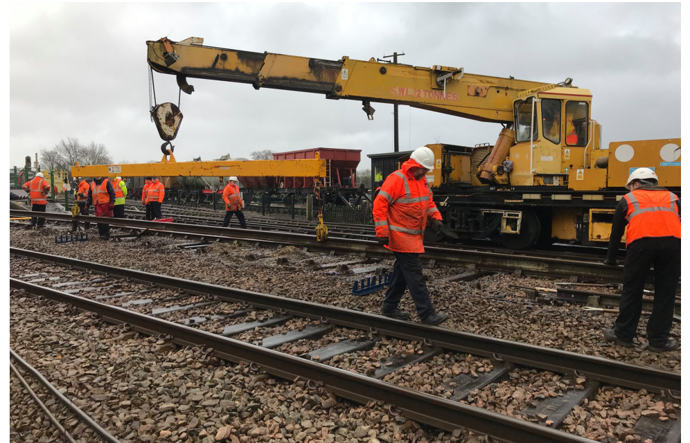
▲ Track Works to replace the sleepers at the south end of Platform 2 during the strong wind and rain of Storm Ciara 9th February 2019 - Peter Robinson
