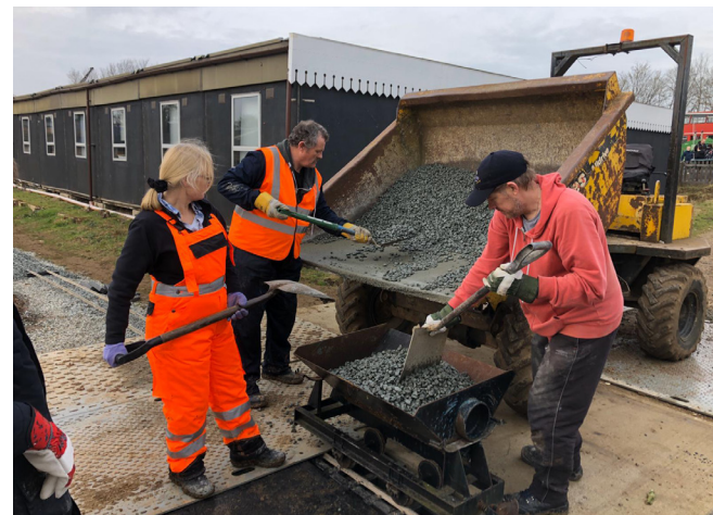
▲ Lesley Pennell, Robert Guest and Niall Thorogood undertake ballasting works on the new Miniature Railway on 26th January 2020 - Tim Rice
