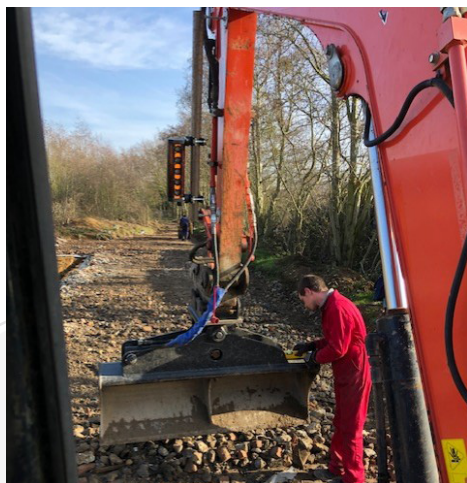
▲ Rob West checking the cross level of the digger bucket for MR2 on 14th February 2019 - Tim Rice.
