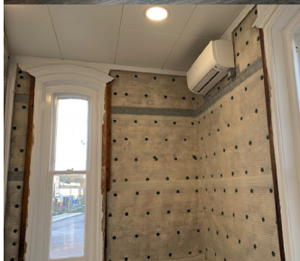
3. Damp proof membrane installed.
