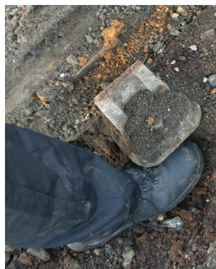
◀ Tallon's boot reveals that there is nothing left of the sleeper once beneath this 1902 check chair.
