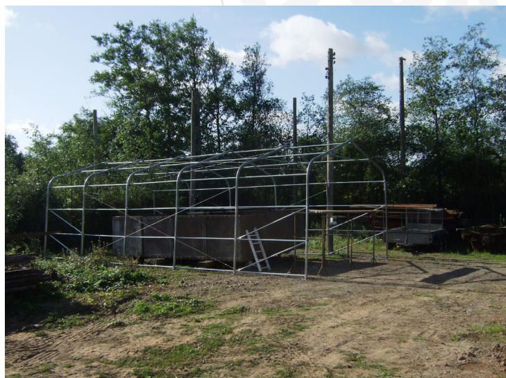
◀ The Frame around the Chelmsford Water Tower, this will be covered and the tank will receive restoration work whilst inside - Mike Stanbury
