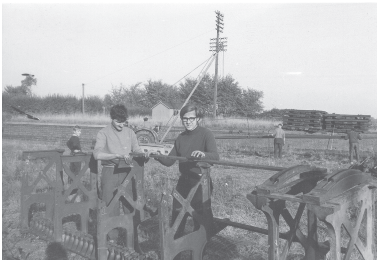
▲ Chris Hunt and Colin Hill re-assemble the signal frame from Chappel signalbox, which was found in the yard, in a badly-damaged state - R Radford. We have included this photo here, as it was intended to be published in Derek Fox's article in SVS163 titled "Episodes of a Heritage Railway Collector" showing the sparse nature of the site in the early days.
