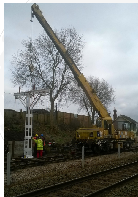
▼ The Signal Gantry being craned into position by the S&T Team - Duncan Reed Tampers supporting the High Output Ballast Cleaner on the GEML reverse at Marks Tey Platform 3 on 15th June 2015 - Darren Johnson ▼
