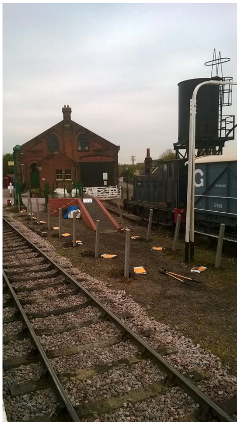
Concrete Sleepers in the track adjacent to Platform 3 and the newly placed fence posts - Duncan Reed
