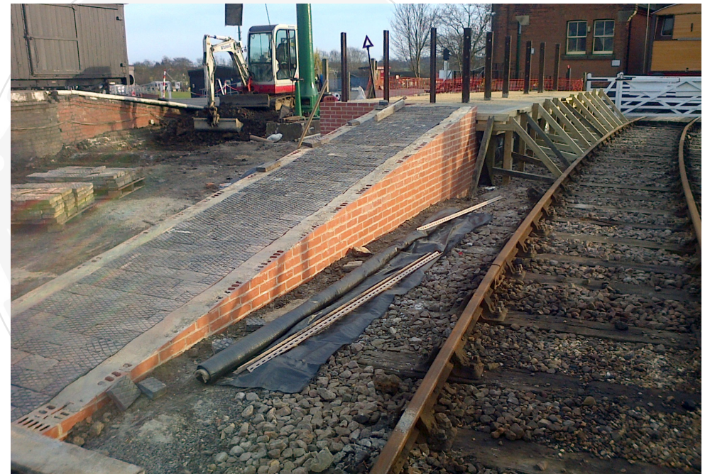
▼ Cattle Dock Ramp and Setts Installed, Prior to Edging Bricks, March 2014 (Ian Reed)
