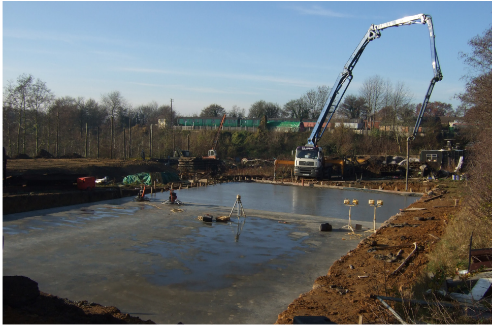
▲ The Concrete Foundations of the Storage Barn being Laid, 11th Dec 13 (David Reeve)
