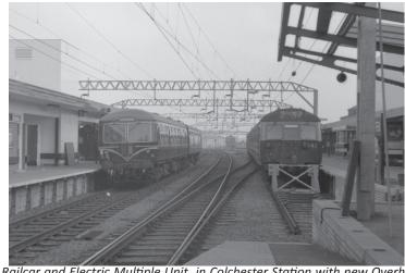
Diesel Railcar and Electric Multiple Unit in Colchester Station with new Overhead Line Equipment
