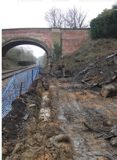
The North Headshunt with the Track Removed. Duncan Reed
