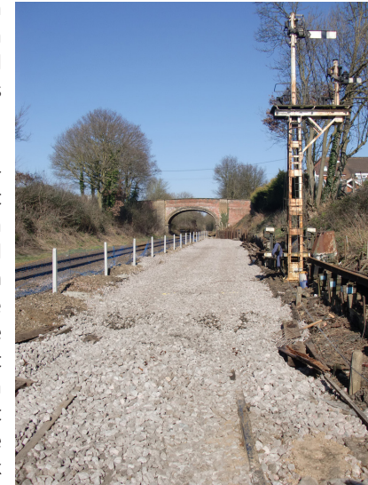
Work Under Way - Fresh Ballast and Fencing before the track is relaid. Rob Boyce
