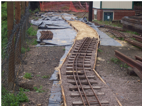
Track extension works on the Miniature Railway
